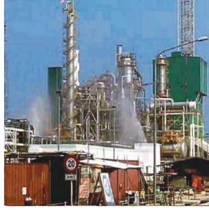
Ammonia Leak in Sabah, 2016
